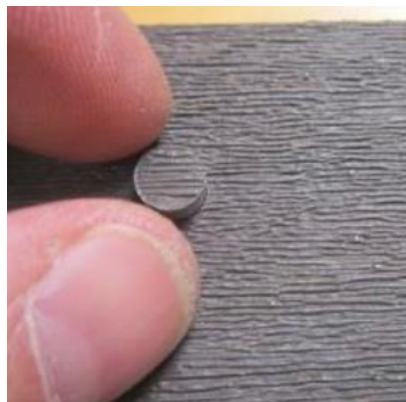
Align the 'grain direction' of the plug and push into hole.
