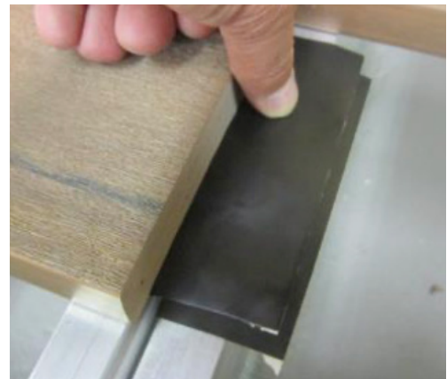
Install appropriate layers of joist tape to shim up the low side.
