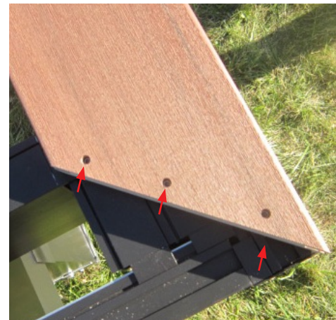
Within \frac{1}{2} " of ends, along miters, and butt-joints
