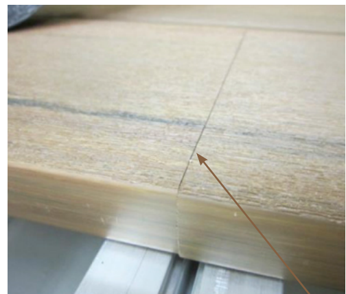
After Joist Tape , joint shows an even flush surface , then fasten down.
