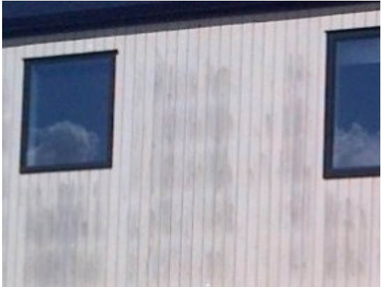
8.5 A New Zealand housing project with a very distinct batten (sub-frame) silhouette showing in the cladding surface
